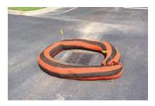
Inlet protection devices, also known as hydrodynamic separators, are flow-through structures with a settling or separation unit to remove sediments, oil and grease, trash, and other stormwater pollutants. This technology may be used as pre-treatment for other stormwater management devices. Inlet protection devices are commonly used in potential stormwater "hot spots"—areas where higher concentrations of pollutants are more likely to occur, such as gas stations.
